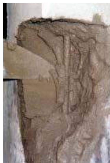
Apply the mortar
