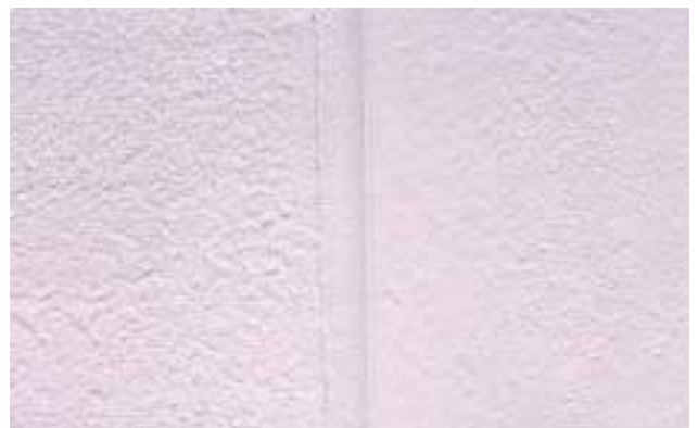
View of the finished joint. It can be painted with the desired colour
