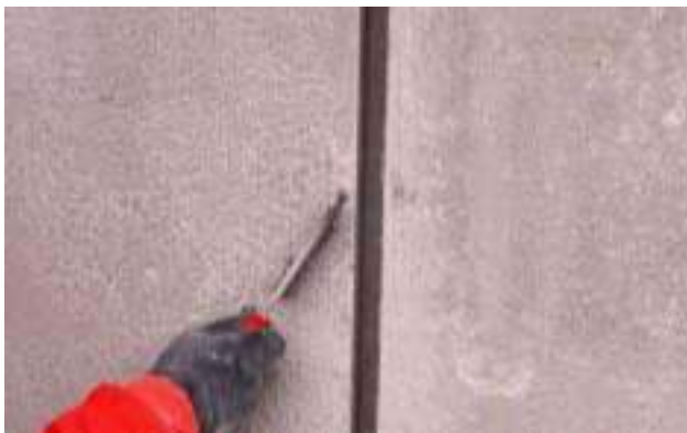
Preparation and cleaning of joint
