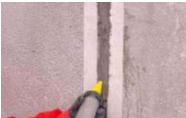
Application of MAXJOINT ELASTIC
